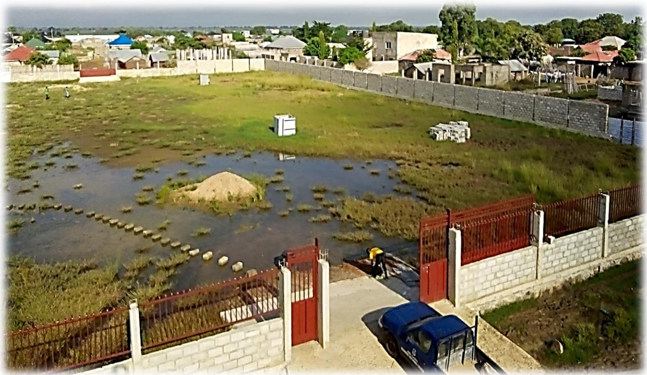
The reclaimed land newly built fence with assistance from Word & Deed
