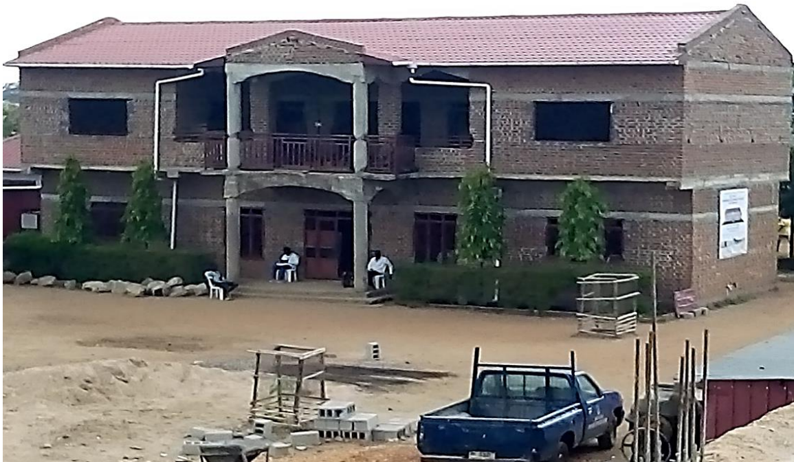
Unfinished SRC Synod Building, Mangateen Juba South Sudan December 2023
