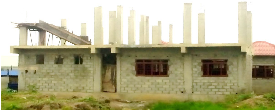
Bethel Secondary School classrooms under construction
