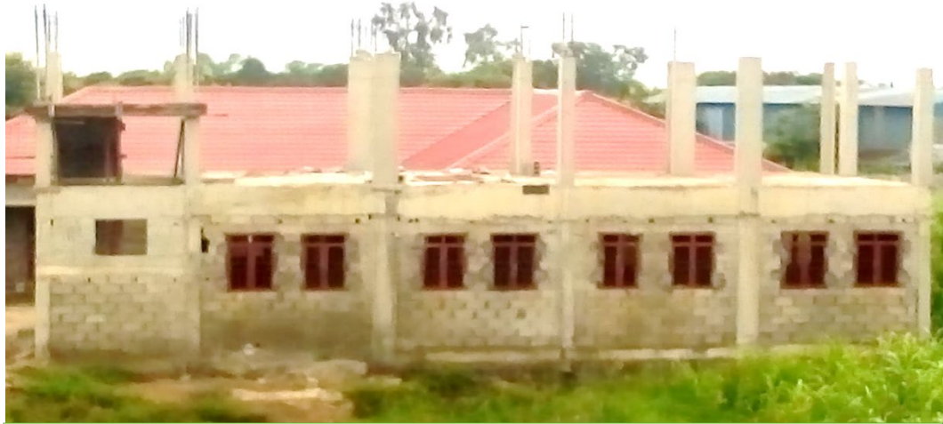
Bethel Secondary School classrooms under construction
