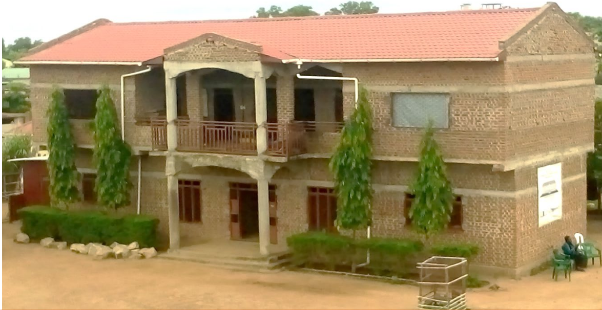
SRC General Synod Office under construction in Juba
