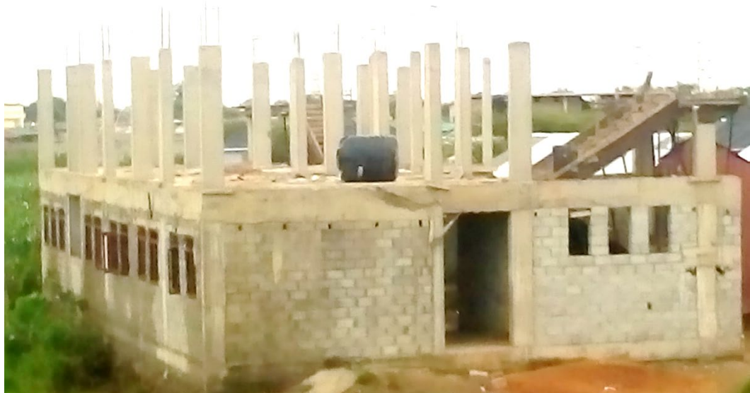
Bethel Nursery classrooms under construction
