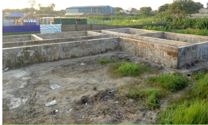
Foundation of Bethel Secondary School, Juba
