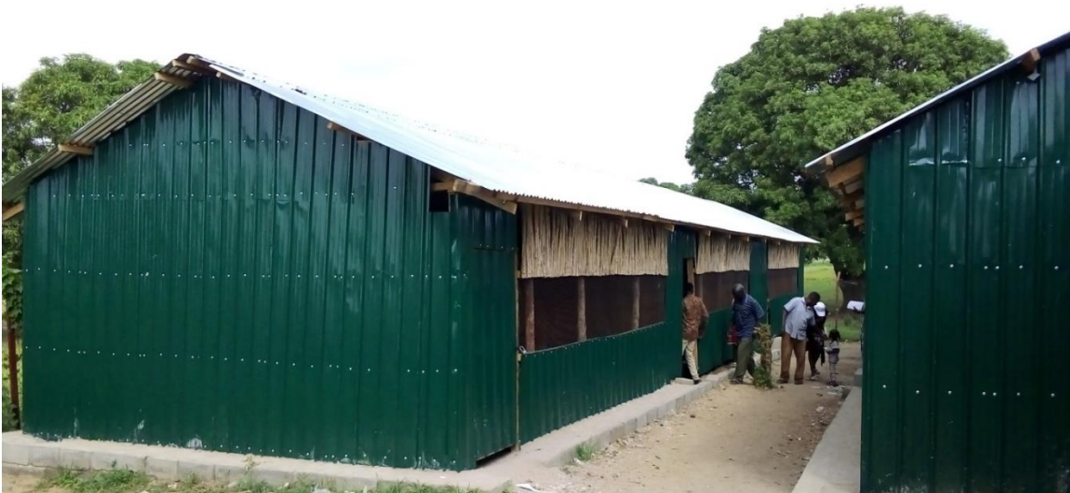
Newly constructed Grace Primary School, Khor Wulyang Juba
