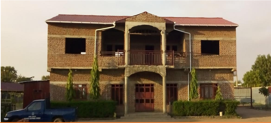
SRC General Synod building under construction
