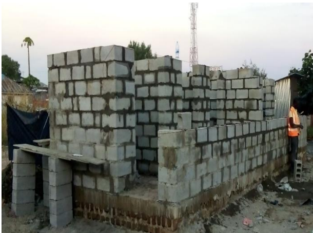
Four stances' toilets under construction, Bethel
